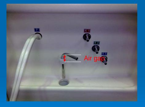
To avoid a retrograde contamination of the dialysis machines from the drain an air gap is strongly recommended
