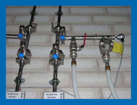
Upon installation stainless steel ring mains can be equipped with additional steam traps and drain fittings.
